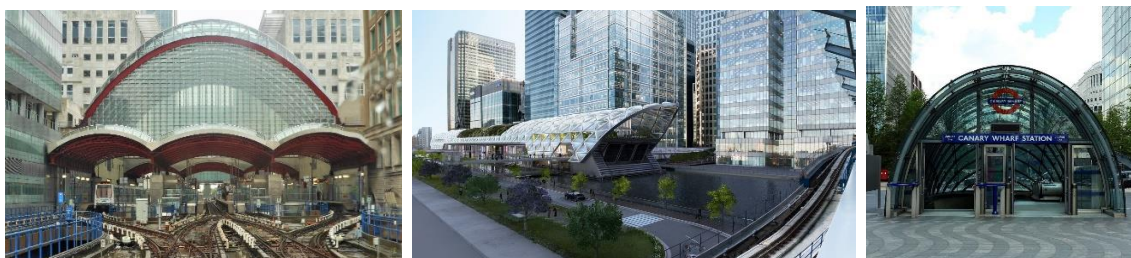
179. Londres, Canary Wharf station.
