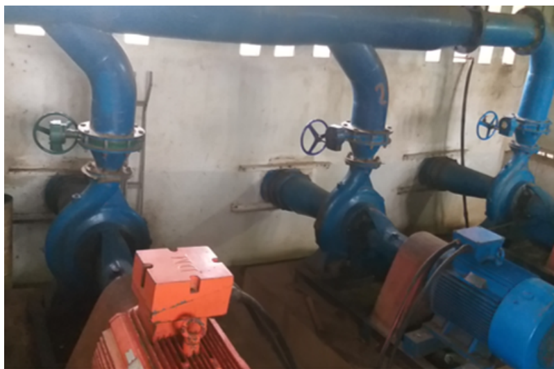
Figure 3.11: Installed pump and motor units.
