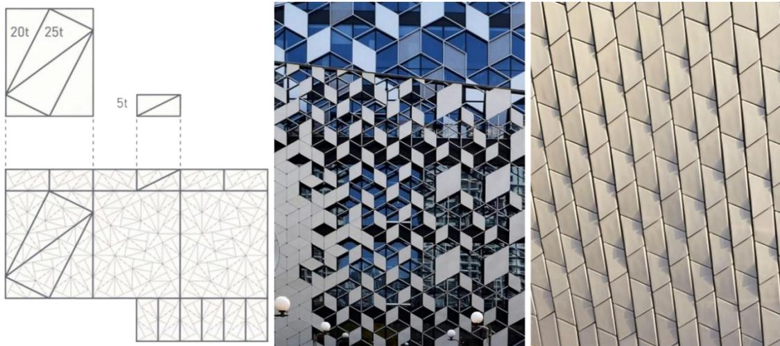
Figure 6.22. From left to right: the triangular tiling rule of the Federation Square facade (edited from [47]); the diamond-shaped facade of Lane 189 (©Eric Jap); MAAT facade tiles (©HUFTON+CROW / AL\_A).
