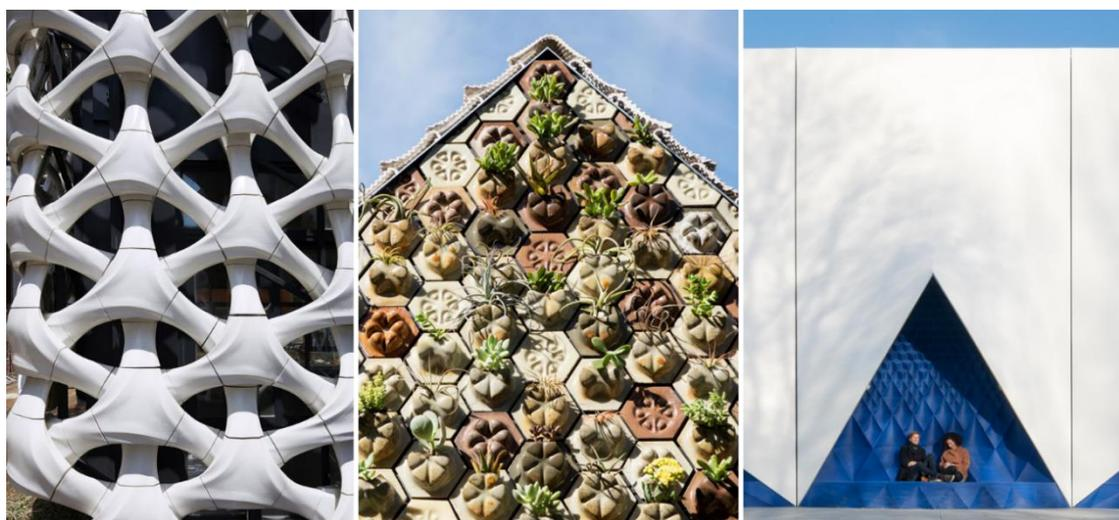
Figure 6.1. Additive manufacturing examples (from left to right): Arachne 3D printed facade by Lei Yu (©Architizer); House of 3D Printed Curiosities by Emerging Objects, 2018 (©Matthew Millman); EU Building 3D printed facade by DUS Architects, 2015 (©Ossip van Duivenbode).
