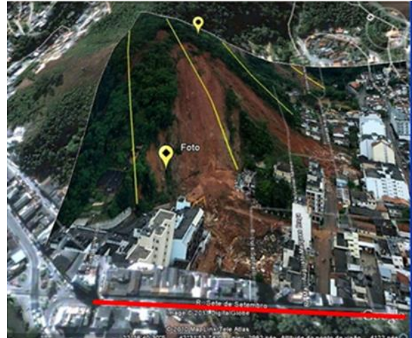
Figure 21: The same area in Nova Friburgo after landslides Source: www.zonaderisco.blogspot.pt
