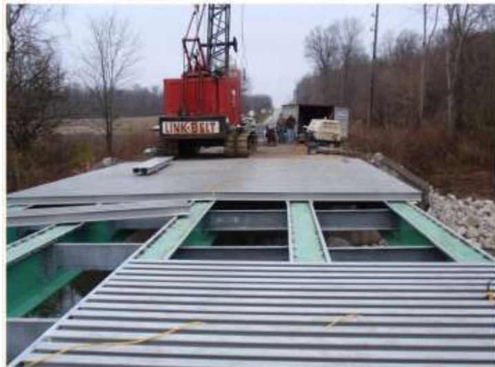
Figure 1.8 - Replacement of a corroded concrete deck with a FRP deck, Indiana 2009. (ZellComp).
