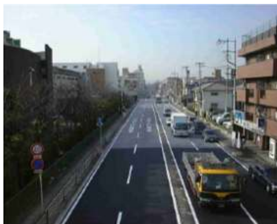
Figure 2.9 - Application of \text{TiO}_2 Highway section (the lighter coloured section of the road) (Fujishima et al., 2008).
