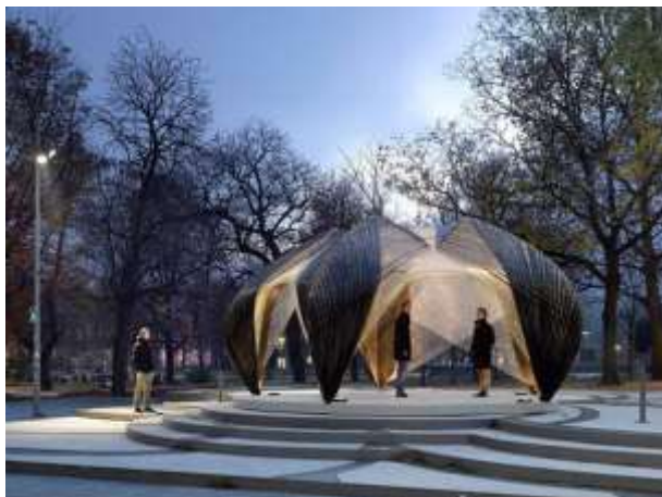
Figure 1.9 - Robotically fabricated pavilion in Stuttgart with carbon and glass FRP. (Evolvo competition, 2013).
