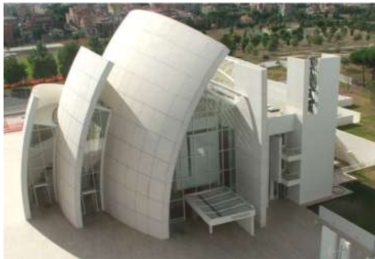
Figure 2.8 - The “Dives in Misericordia” church, constructed of \text{TiO}_2 -containing self-cleaning cement (Pacheco-Torgal and Jalali, 2011).
