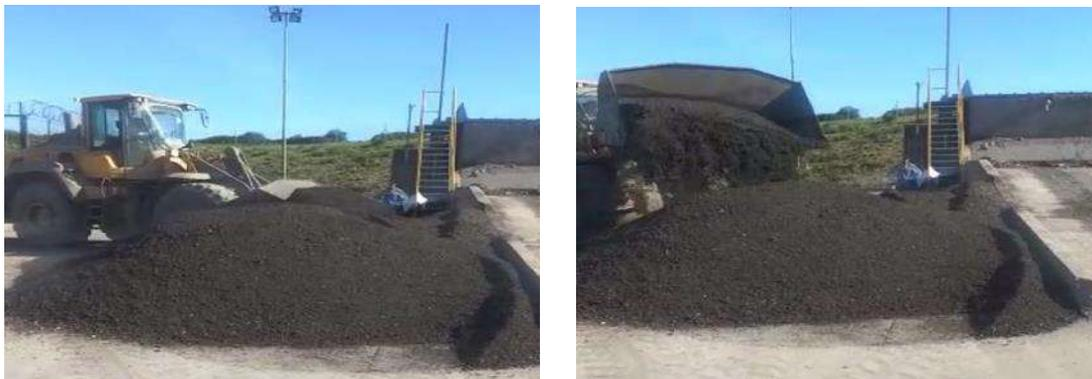
Figure 2 - Homogenization of MIBA
