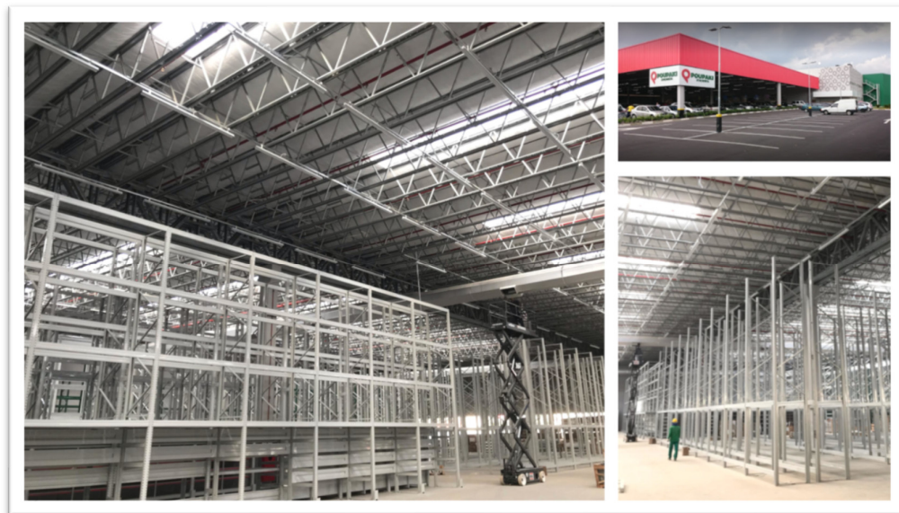
Figure 1.1. Roll-on roofing system from MARKO Sistemas Metalicos, consisted of cold-formed steel members, illustrated in the construction of Poupaki wholesaler, located in the city of Guarulhos, São Paulo, Brazil [4].
