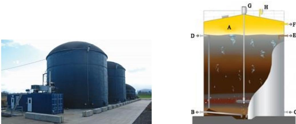
**Fig 9.** Representation of the Clearcove digestion systems and the anaerobic digestion system: A) Biogas enclosure; B) Ground sludge pipe; C) Ground injection pipe; D) Substrate inflow; E)
