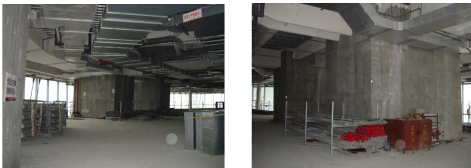
Figure 4.12 - A pair of super-columns on the 60th floor
