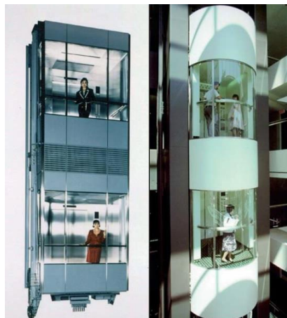
Figure 4.47 - Double deck elevator (Russett, 2010)
