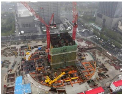
Figure 4.17 - Shanghai Tower – Concrete core construction in December 2011 (JKEC, 2012)
