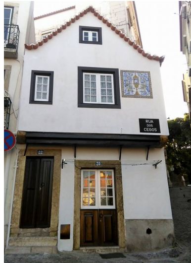
Figure 2-33 - Building with “ressalto” floors
