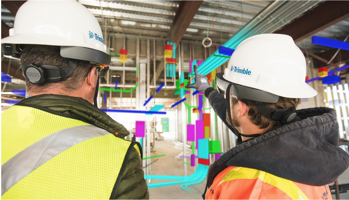
Figure 2.4: AR application in MEP, where 2 technicians wearing AR goggles are able to see, in fluorescent colours, a virtual representation of MEP elements in their precise future location (from [20]).
