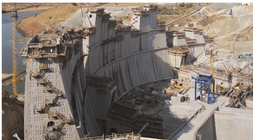
Fig. 3.8 Alqueva dam during construction. View of a contraction joint with shear keys of hemispherical shape.
