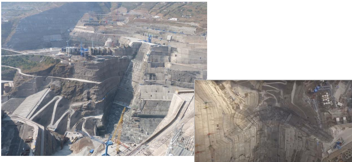
Fig. 2.16 Aerial view of the foundation of Baihetan dam (China) in 2017, before construction. Insertion surface.
