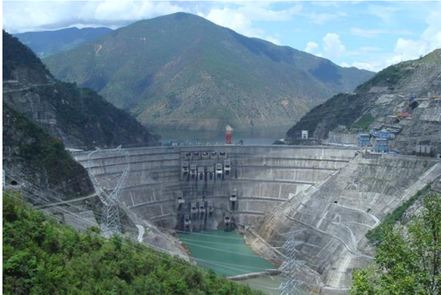
Fig. 2.5 Arch dam: Xiaowan dam (2010), China, 292 m high.
