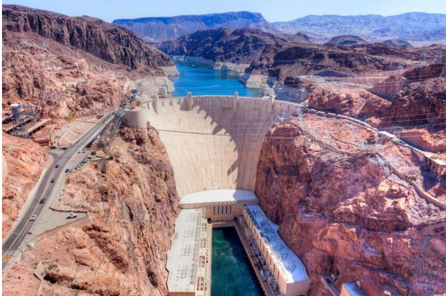
Fig. 2.7 Arch-gravity dam: Hoover dam (1936), United States of America, 225 m high.
