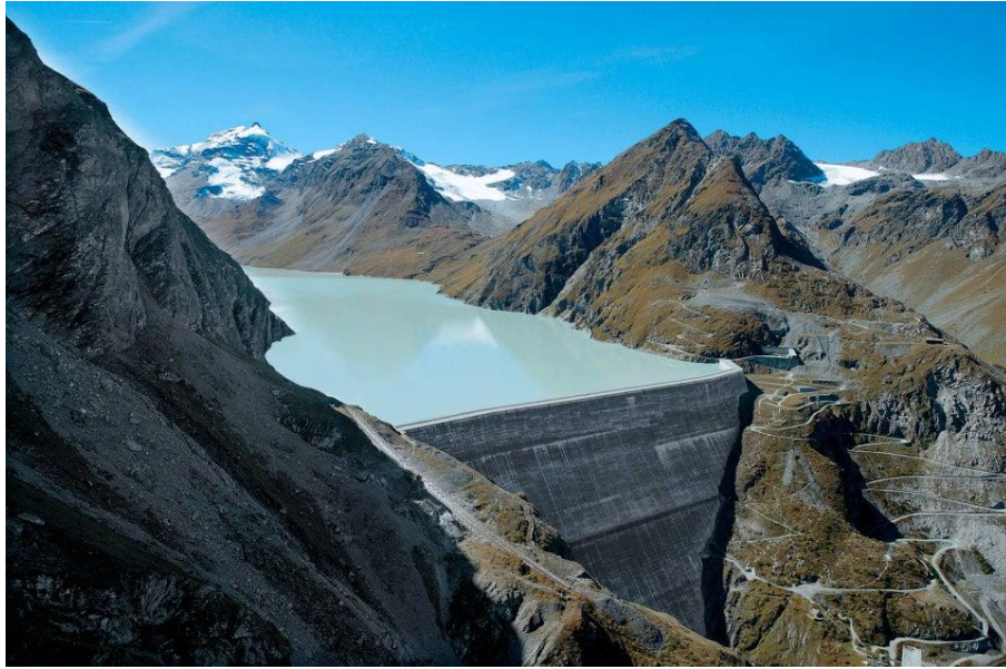
Fig. 2.2 Gravity dam: Grande Dixence dam (1961), Switzerland, 285 m high.
