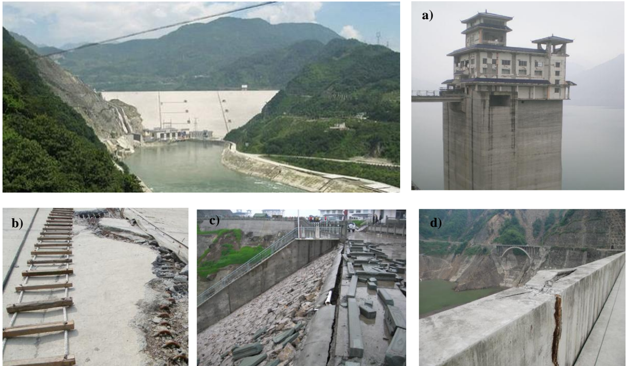
Fig. 2.29 Zipingpu concrete face rockfill dam, 156 m high, China. Consequences of the 2008 Wenchuan earthquake: a) damaged structure on top of the intake tower; b) damage along vertical joints on the concrete upstream face; c) damage on the downstream face and gap between the stone masonry and the crest; and d) crack at the crest.
