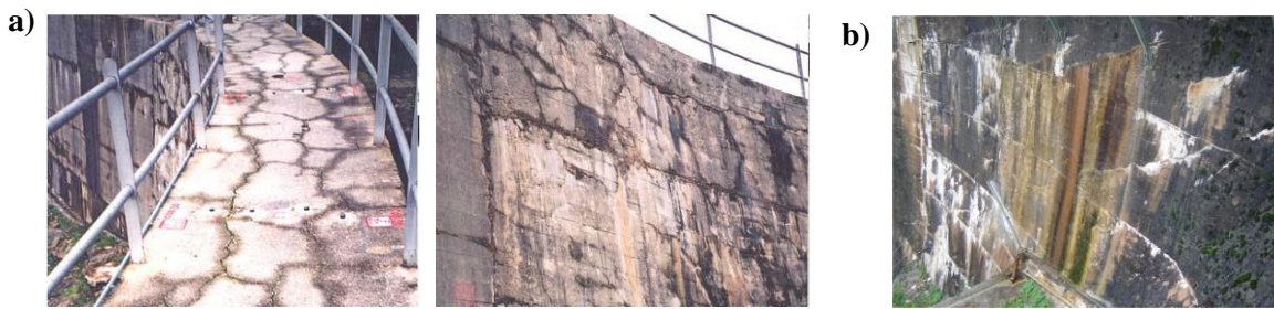
Fig. 2.18 Old Alto Ceira I dam (1949), Portugal, 34 m high. a) Cracking at the crest and on the downstream face; b) Signs of water percolation through joints/cracks and products of swelling reactions (Batista & Piteira Gomes, 2014).
