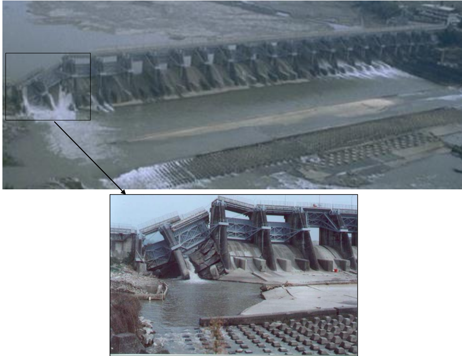
Fig. 2.28 Shih-Kang weir, 25 m high and 352 m long, Taiwan. Failure of two openings, close to the right bank due to fault movements during the 1999 Chi-Chi earthquake.
