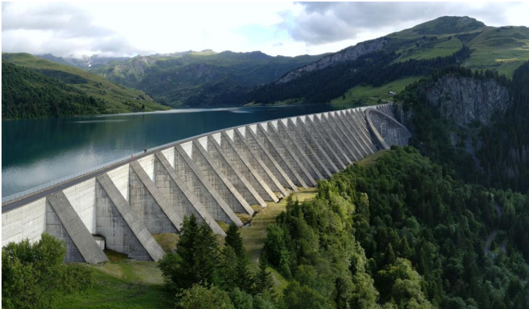
Fig. 2.4 Buttress dam: Roselend dam (1962), France, 150 m high.
