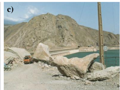
Fig. 2.27 Sefid Rud buttress dam, 106 m high, Iran. Damages during the 1990 Manjil Earthquake: a) crack at the top of the upstream face; b) crack at the kink of a buttress (downstream face); and c) access roads blocked by rockfalls.
