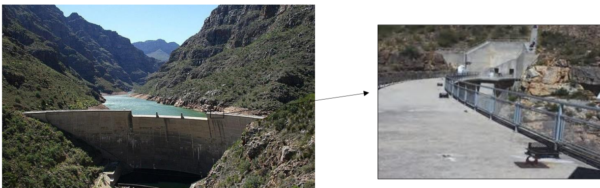
Fig. 2.54 Roode Elsberg dam, South Africa. Downstream view and location of the installed accelerometers in December 2013 (Bukanya, 2020).
