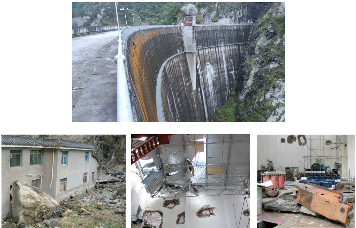
Fig. 2.30 Shapai RCC arch dam, 132 m high, China. Consequences of the 2008 Wenchuan earthquake: effects of rockfalls on the powerplant and damage equipment inside the powerhouse.
