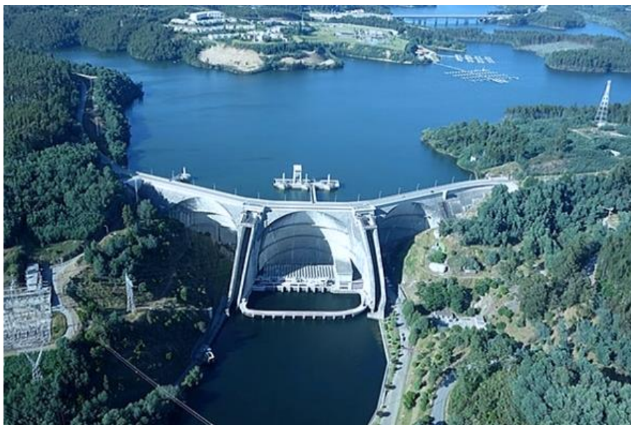
Fig. 2.8 Multiple-arch dam: Aguieira dam (1972), Portugal, 89 m high.
