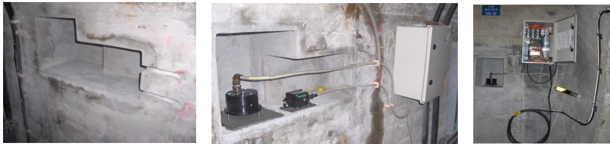
Fig. 4.7 Installation of the dynamic monitoring system at Cabril dam. Uniaxial and triaxial accelerometers, equipment storage box for data acquisition units, and optical-fibre cables (S. Oliveira & Silvestre, 2017).
