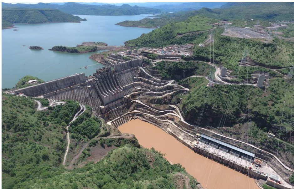
Fig. 2.3 Roller-compacted gravity dam: Gilgel Gibe III dam (2015), Ethiopia, 250 m high.
