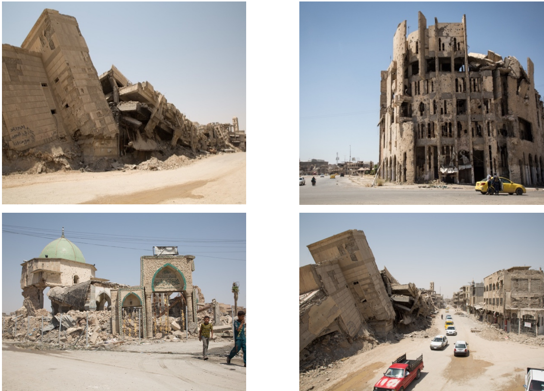
Figure 86. Local authorities helped the local people clean some main streets’ rubble (Source: author).
