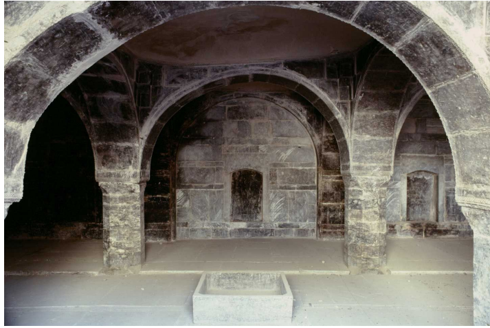
Figure 37. The use of marble in the basement of a traditional house in Mosul (Source: Mosul Eye).
