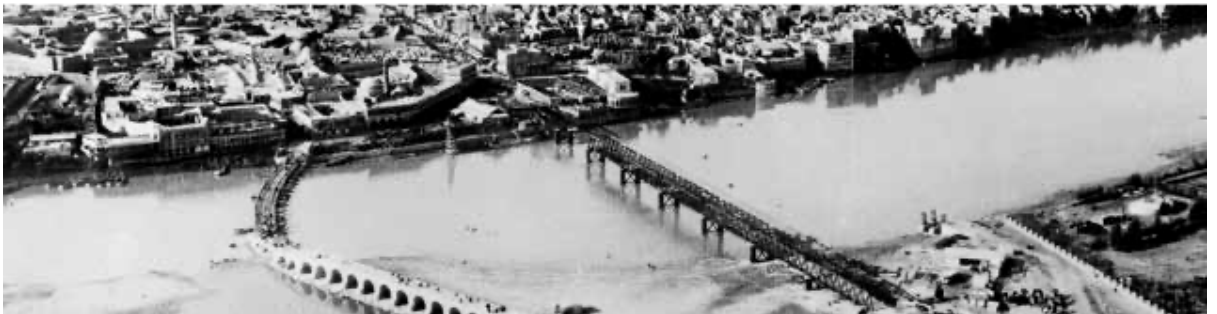
Figure 15. Mosul's old and new bridges, 1933- 1934 [24].
