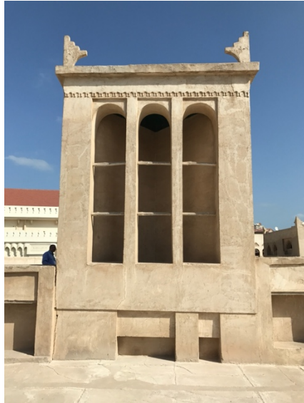
Figure 33. An example of Wind tower (Malqaf) (Source: author).
