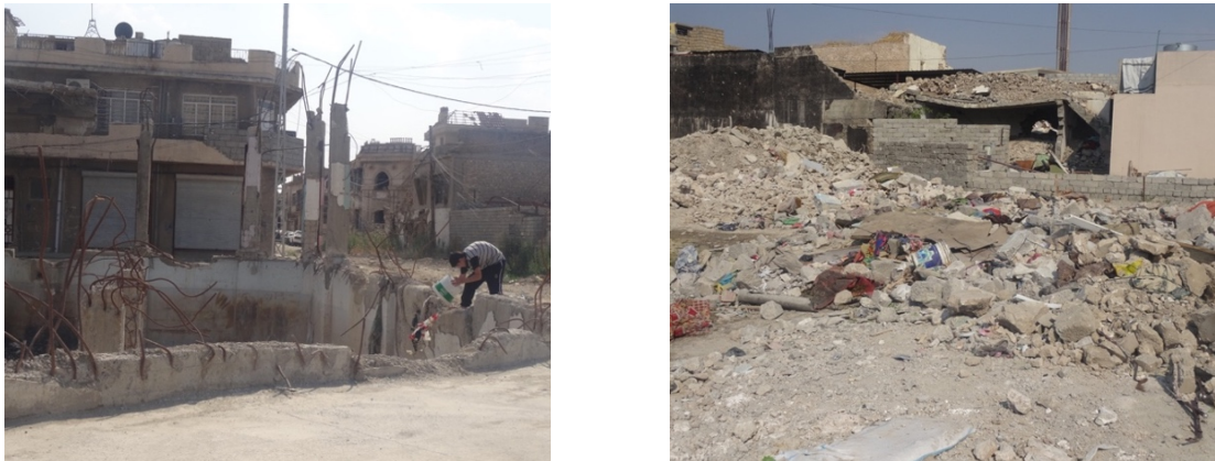
Figure 90. Mixed rubble with household waste in western Mosul (Source: author).
