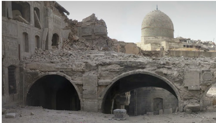
Figure 35. Al Tutunji house after destruction (Source: Iraq Heritage Stabilization Program).
