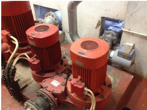
(c) BPC2 - pumps water into the Small Chiller.
