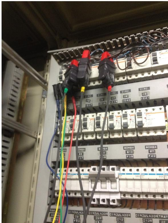
Figure 4.12: Chauvin connected to the electric panel - electric panel of the Garage Technical Area of the IST Alameda Campus Civil Engineering Building.
