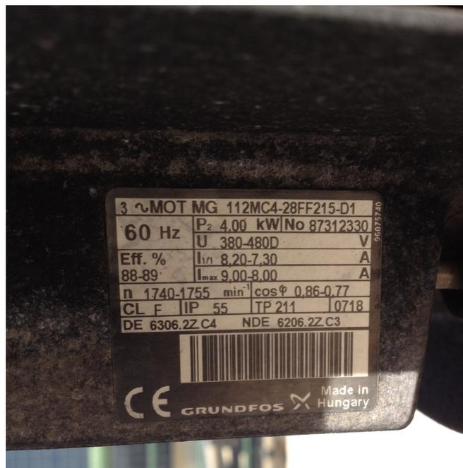
Figure 4.1: Example of a three-phase induction motor nameplate - motor of a pump located on the rooftop of the IST Alameda Campus Mathematics Building.
