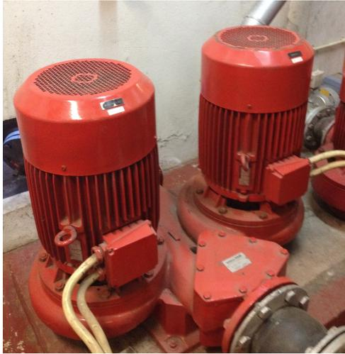
(a) BPC1 - pumps water into the Big Chiller.
