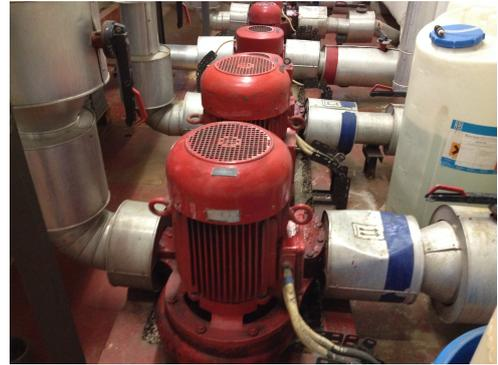
(b) BF1 - pumps water into the cold water circulation system.
