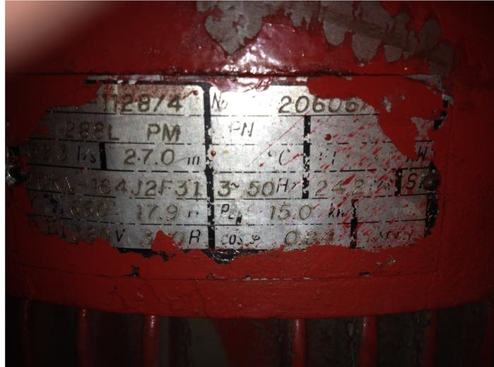
Figure 4.2: Example of an induction motor unreadable nameplate - motor of a pump located on the Cold Central of the IST Alameda Campus North Tower.
