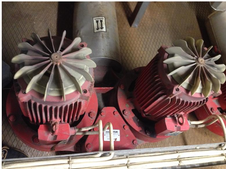
(e) BQ1 - pumps water into the hot water circulation system (cooling fan protections are off the motors in order to allow direct contact speed measurement using the tachometer).
