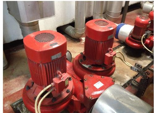
(d) BPF1 - pumps water into the cold water circulation system.
