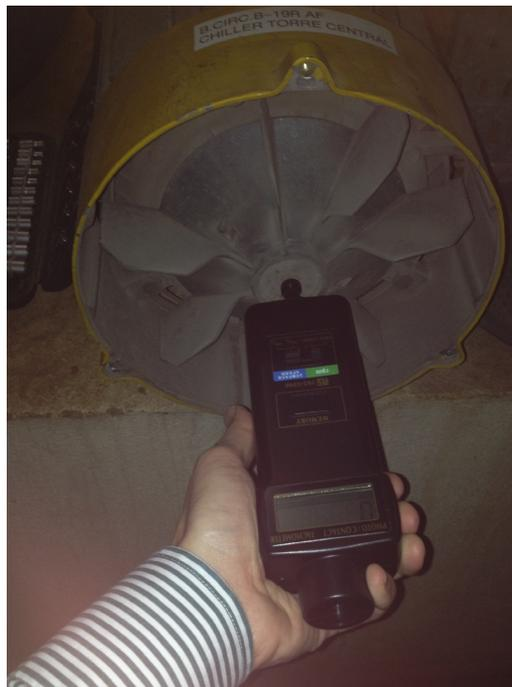
Figure 4.14: Motor speed measurement by direct contact using the tachometer - motor of a pump of the Garage Technical Area of the Alameda Campus Civil Engineering Building.
