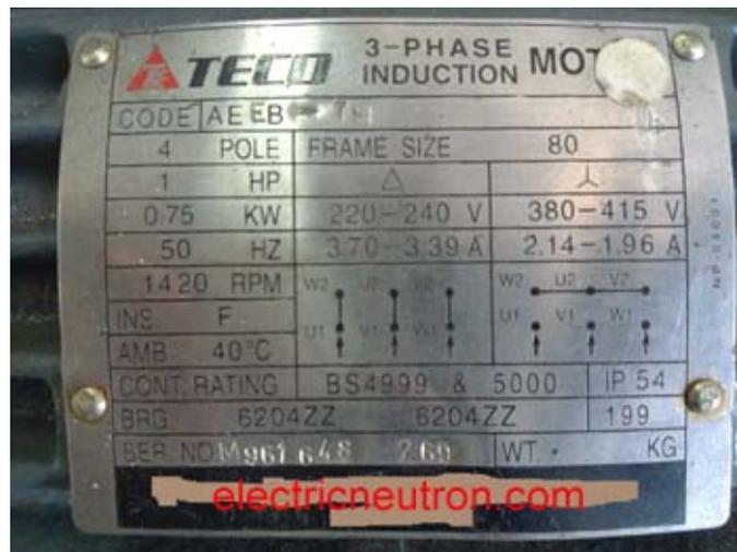
Figure 4.4: Example of a three-phase induction motor nameplate with star and delta connections information [electricneutron.com, 2017].
