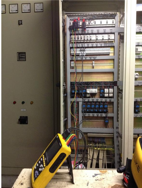
Figure 4.11: Chauvin retrieving data over time - Garage Technical Area of the IST Alameda Campus Civil Engineering Building.
