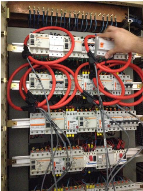
Figure 4.10: Fluke connected to the electric panel - electric panel of the Cold Central of the IST Alameda Campus North Tower.
