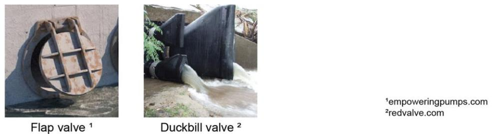
**Figure 3-4.** Examples of tidal valves
