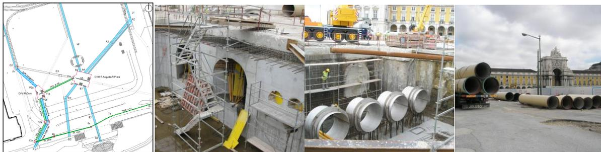
**Figure 6-12.** Schematics (HIDRA, 2008) and photos of the construction works of the combined flow control chambers and wastewater interception strategy in Terreiro do Paço (photographs kindly provided by HIDRA)
