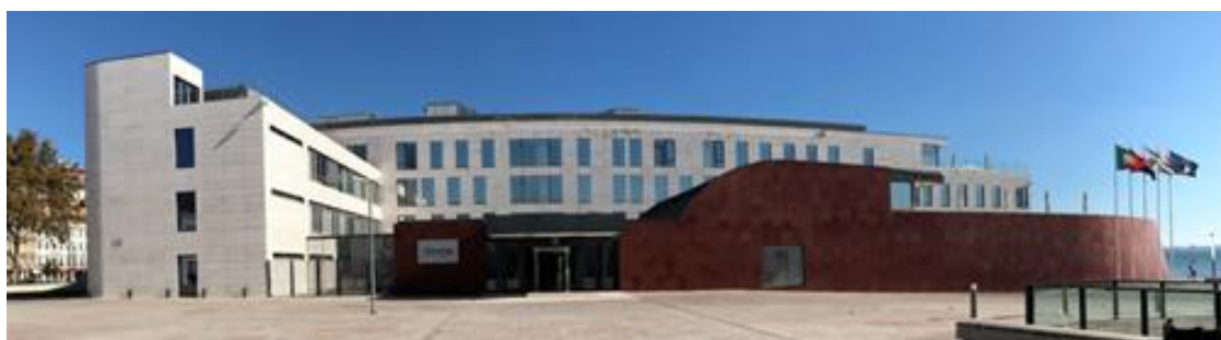
Figure 45. External view of the building of the case study – main entrance
