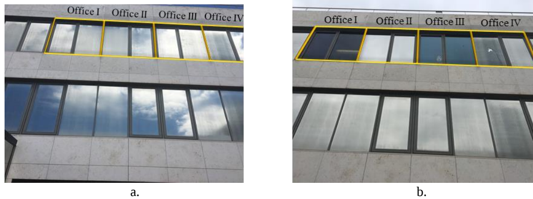
Figure 51. Monitored offices (outer view) before (a) and after (b) the installation of the films
