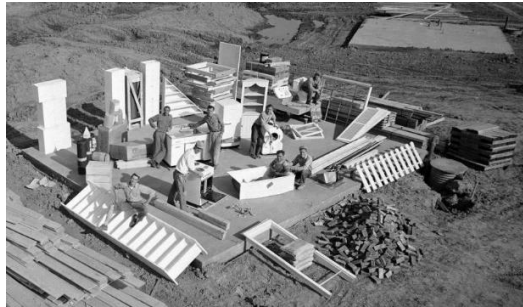
Fig. 99 - Kit de partes em Levittown, 1948 ( http://tigger.uic.edu/~pbhales/Levittown.html ).
