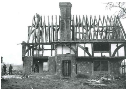
Fig. 28 - Desmontagem de uma "Wealdon house" ( http://www.wealddown.co.uk/images/stories/magazines/2000s/2007%2004%20WDOA%20Magazine.pdf ).
