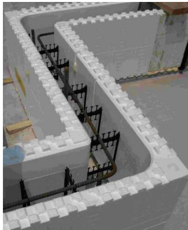
Figure 3.8 - Insulated Concrete Forms (ICF) (R&R, 2011)
