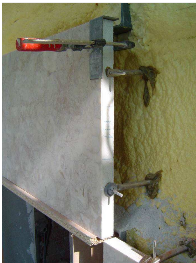
Figure 3.12 - Ventilated rainscreen façade - detail of the fastening system of a natural stone cladding
