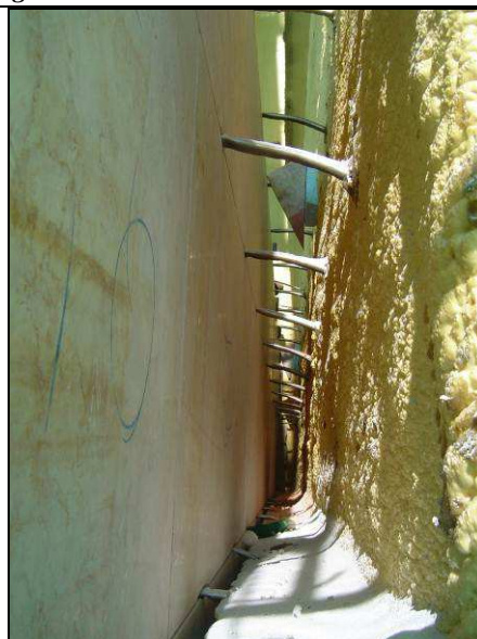
Figure 3.13 - Ventilated rainscreen façade - view of the lower part of the façade with the “mortar bed” for water drainage and opening for ventilation
