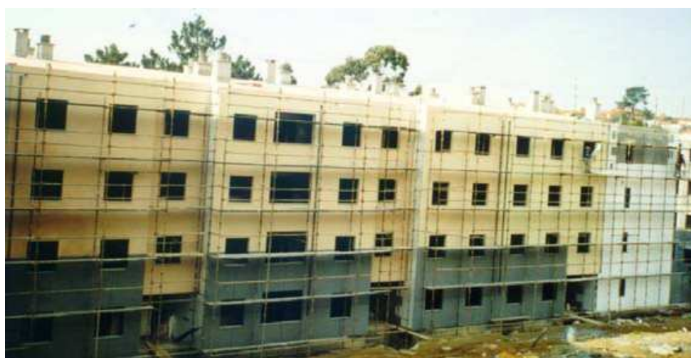
Figure 3.10 - ETICS applied in a building in Lisbon, Portugal (Veiga, 2004)
