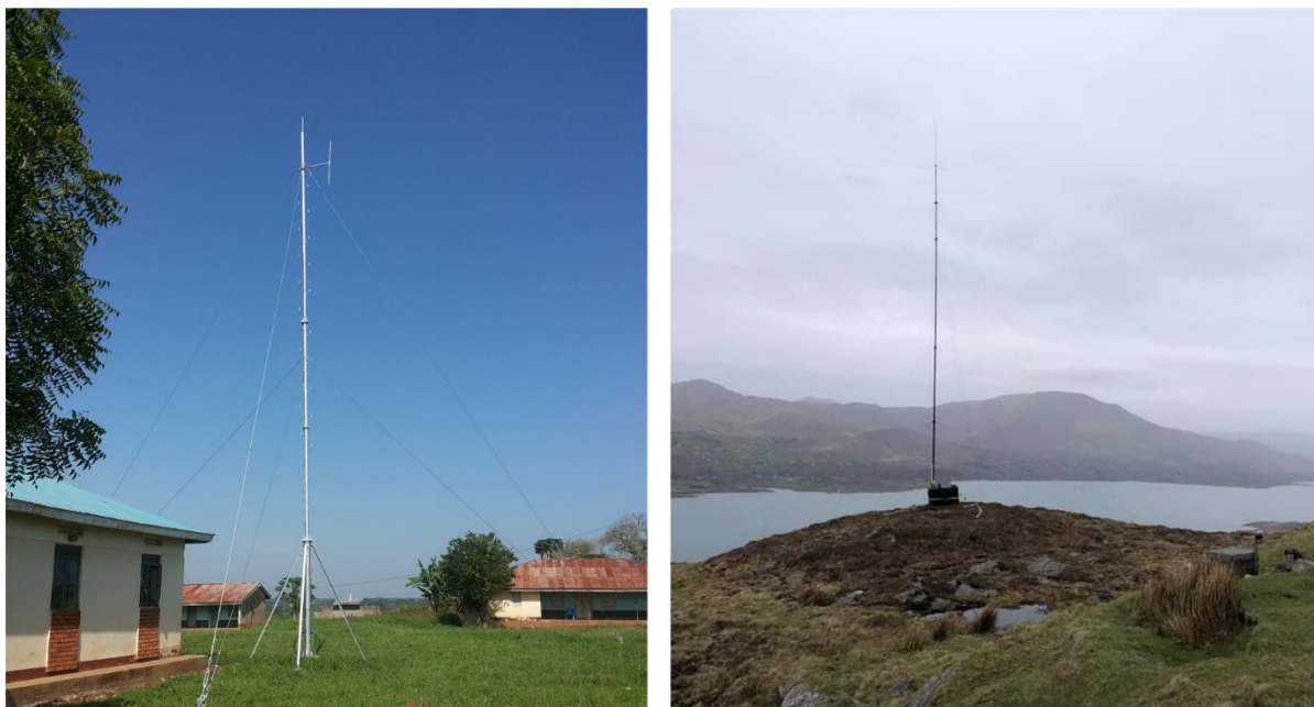
Figure 3.5. Images showing a steel tower with side mounted T-shape dipole antenna in Uganda (left) and fiberglass antenna with top mounted monopole antenna with ground plane in Ireland (right)
