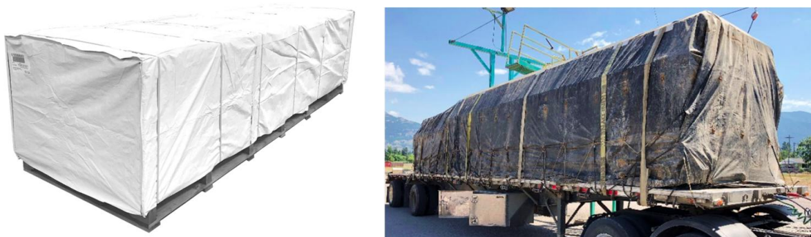
Figure 43. Temporary protection against weather conditions (SmartLam, 2020)
