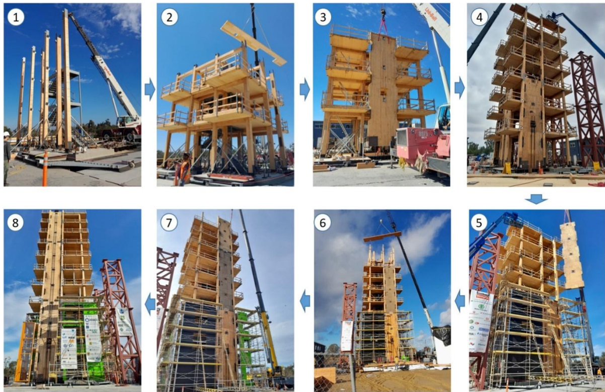
Figure 66. Structural construction sequence of the test building of NHERI Tall Wood project (Pei et al., 2024)
