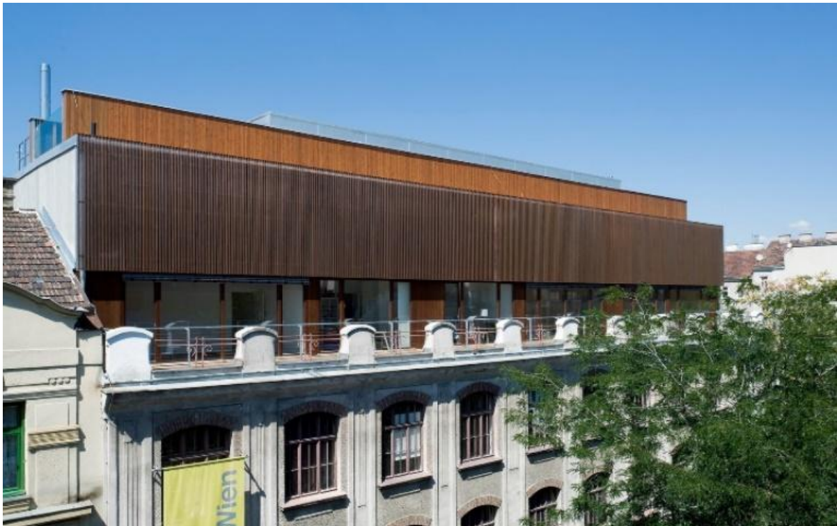
Figure 3. Example of the extension of the existing building with a timber structure (Dietrich Untertfaller Architekten, 2007)
