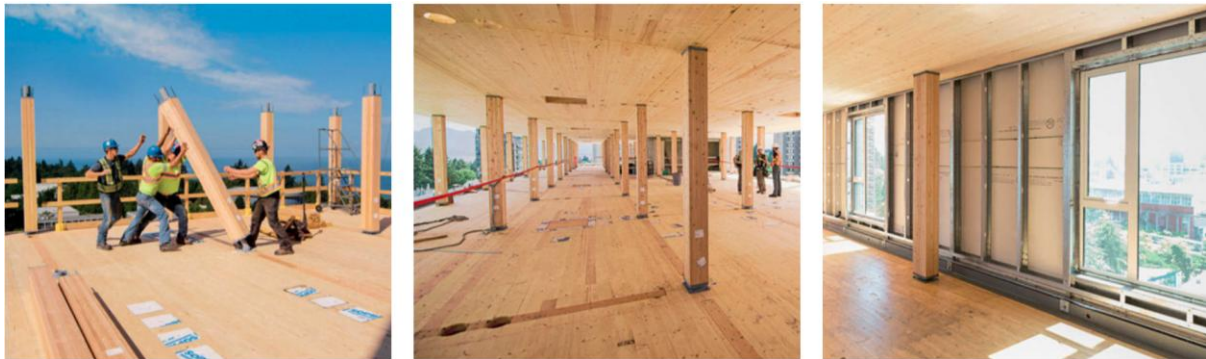
Figure 41. Assembly of prefabricated elements in Brock Commons, two new storeys added each week (Kaufmann et al., 2018)
