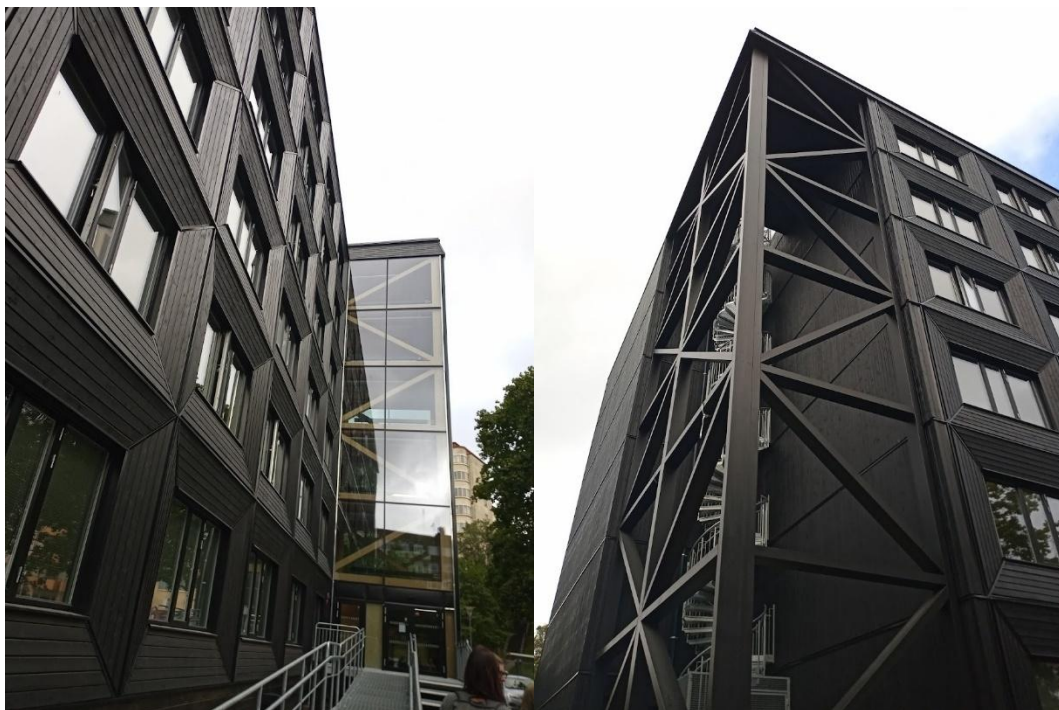
Figure 30. Gibraltar Guesthouse - Modular timber boxes building in Gothenburg
